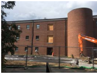
An exterior modification on the south side of WorriLOW Hall is done to make way for a new glassed-in stairwell. The fourth photo illustrates Dean Rieger's remarks regarding demolition of the interior.
