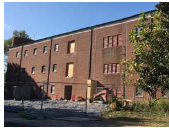
An exterior modification on the south side of WorriLOW Hall is done to make way for a new glassed-in stairwell. The fourth photo illustrates Dean Rieger's remarks regarding demolition of the interior.
